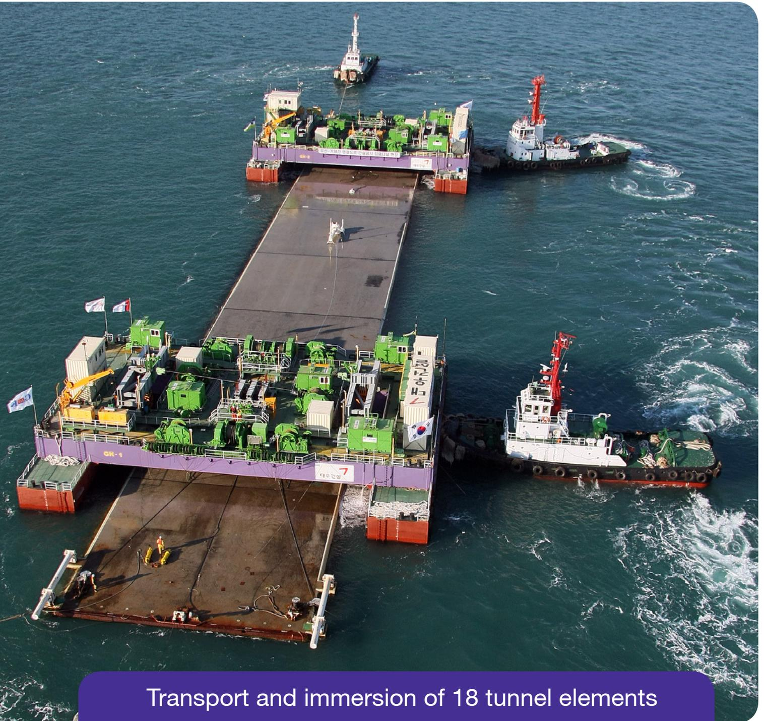
Transport and immersion of 18 tunnel elements
